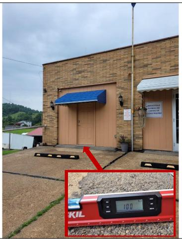
The front entrance is not accessible due to the excessive slope of the parking facility and door threshold. Utilize another entrance that may better comply with ADA Standards; There is a side entrance in compliance with ADA Standards with a paved area in the rear of the building that could be used for accessible parking spaces if marked appropriately.
