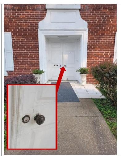
Replace the inaccessible door hardware with a loop, push, or pull hardware. Adjust existing parking signage to the appropriate height requirement (60") and designate at least one space to be van accessible. Install access aisles, complying with ADA Standards 502.2.
