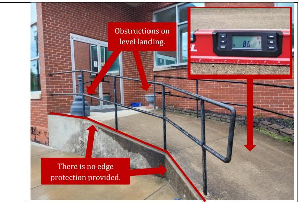
Install handrail extensions and edge protection on the ramp. Ensure the ramp has a level landing, measured 60" by 60", provided at the bottom where it meets the curb ramp. Though there is still a 60" by 60" clearance on the level landing at the top of the ramp, the debris could cause obstruction to entry and should be removed.
