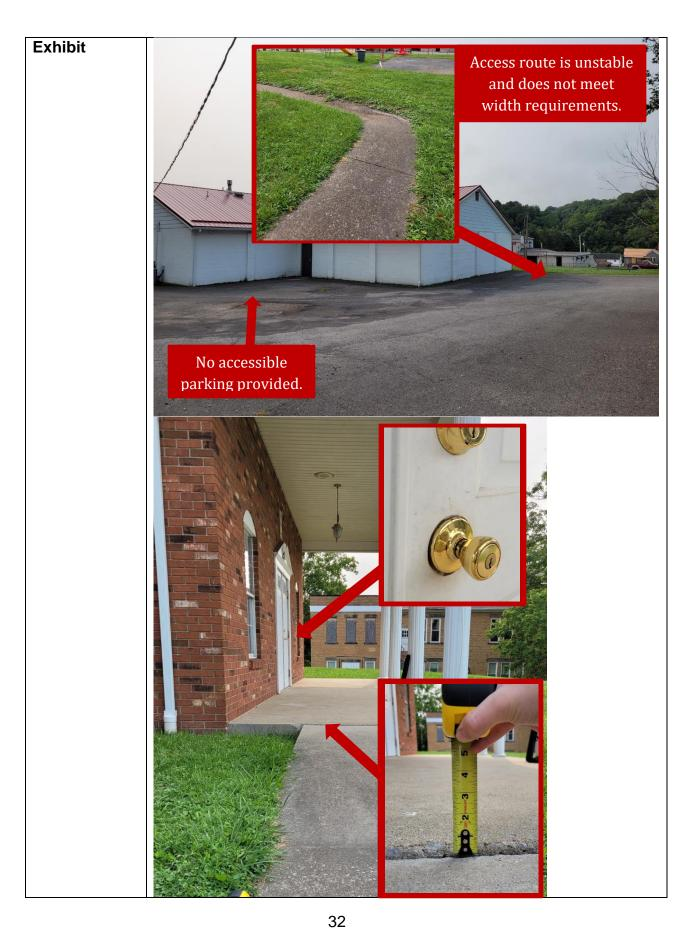
Replace the inaccessible door hardware with a loop, push, or pull hardware. Install at least one van accessible parking space with an access aisle and appropriate signage. Utilizing mats may be an option to extend the width of the access route and cover the crack in the sidewalk, so long as they form a stable surface.
